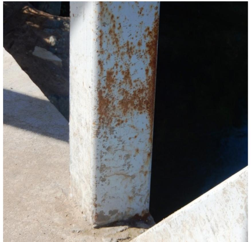
Financial support can help prevent damage by coating the bridge with rust-inhibiting paint
